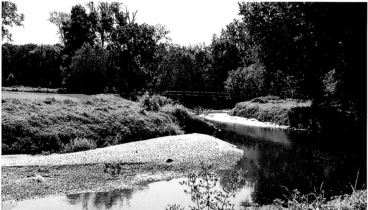
Photograph 4 – Site 3: 12 th Green Bridge and Channel Scour
