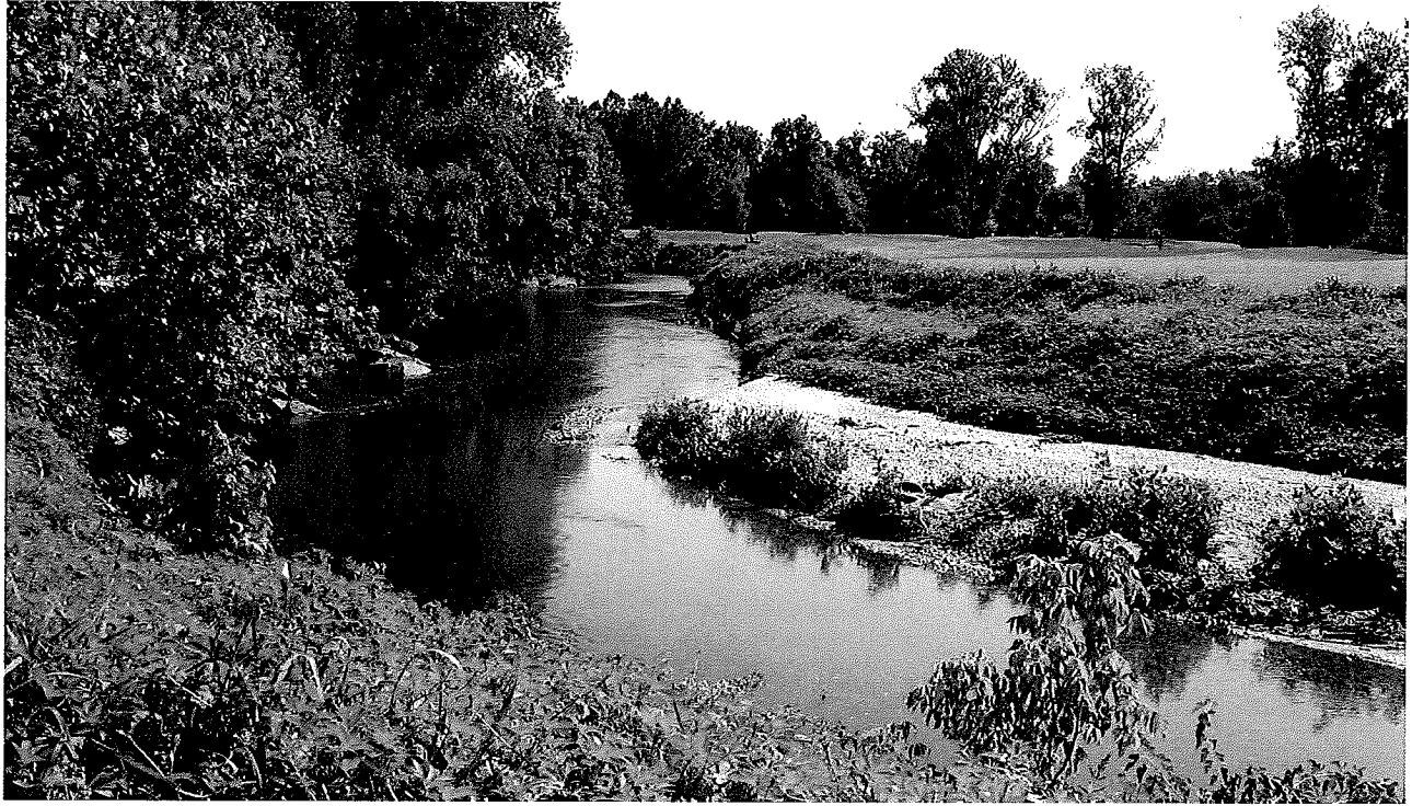
Photograph 5 – Site 4: 12 th Fairway Bank Erosion
