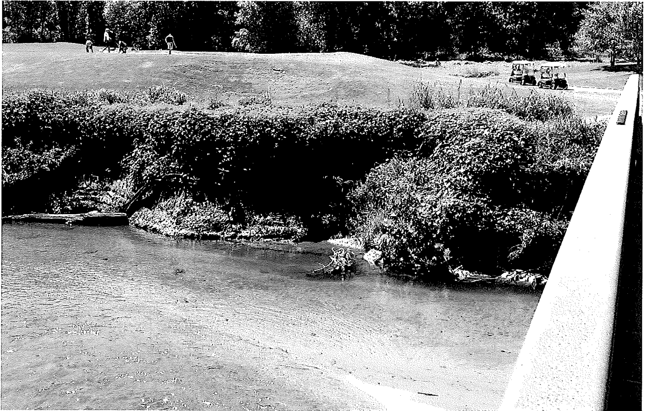
Photograph 7 – Site 5: 11 th Green/2 nd Bridge heading to Hole 3
